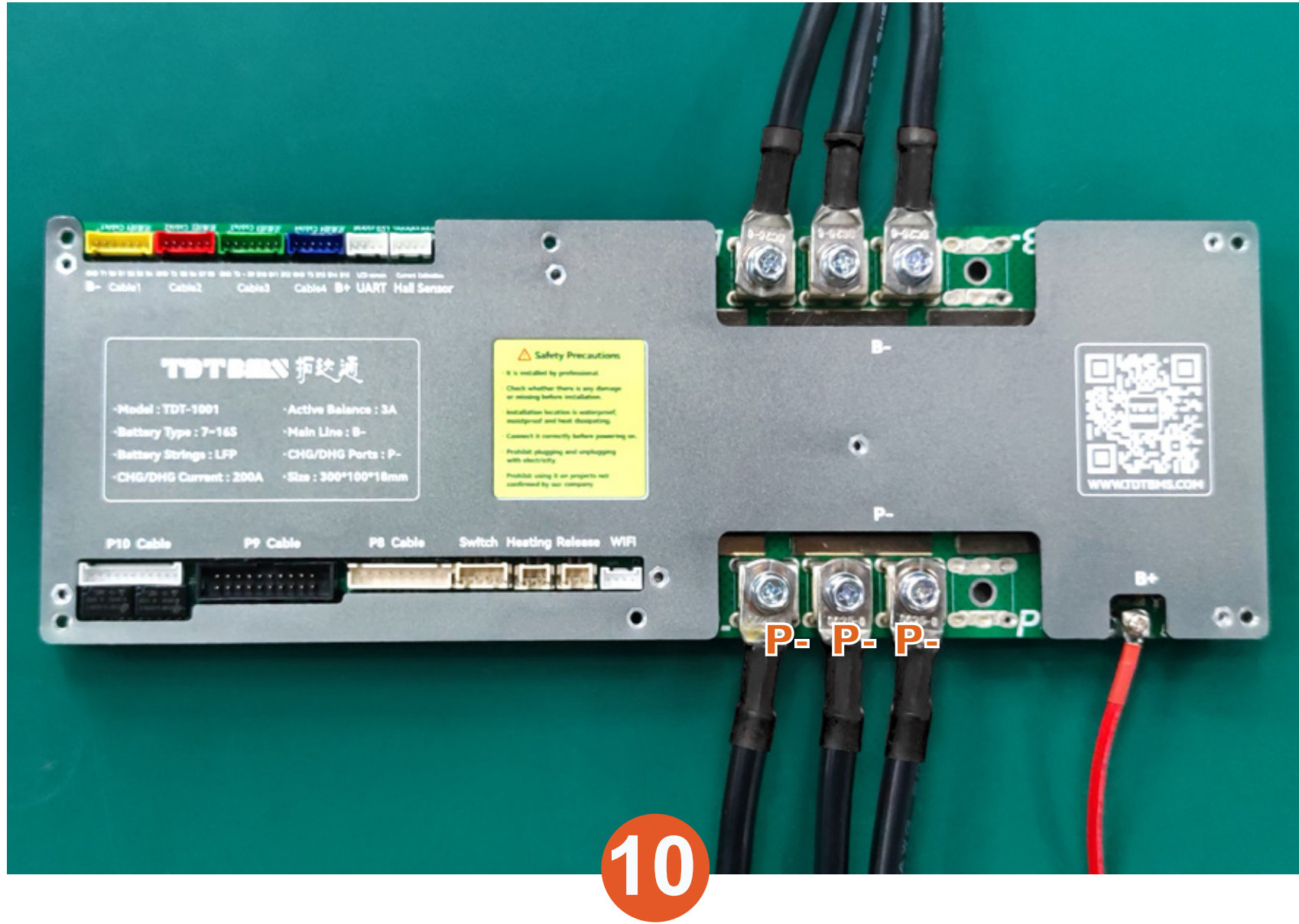
Connect the P- end on the BMS to the negative end of the inverter and charger load with thick silicone wires.
